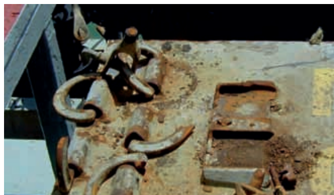
Wasted container securing fittings
